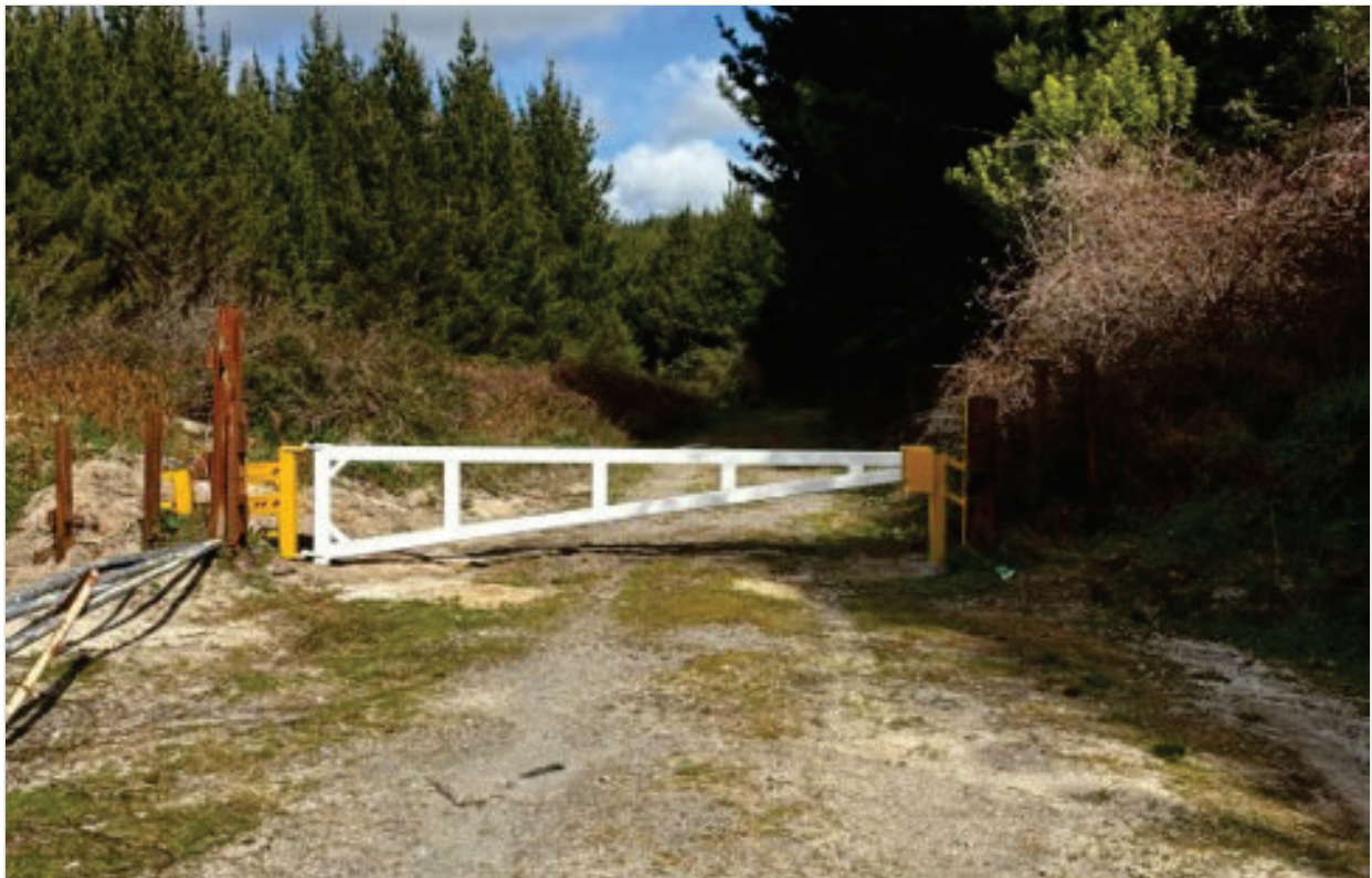
The new entrance gate, closed
